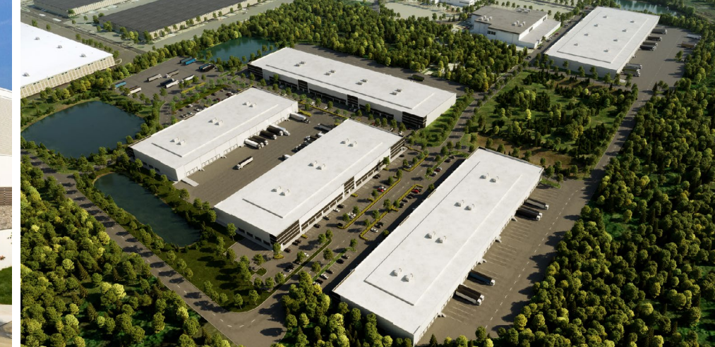
Northlake II 5-Building, 655,000 SF Industrial Park
